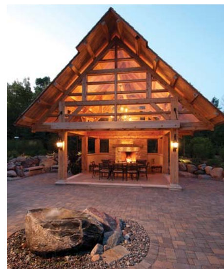
TOP: A spacious terrace, ringed by large boulders, extends the outdoor living area beyond the more protected refuge the gazebo offers. ABOVE: Gable-end windows bring lots of light into the sheltered structure while keeping the gazebo more insulated than a totally open design would allow.
